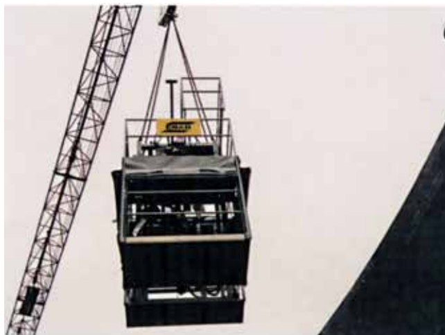
Double-side Circotech being lifted onto the job.
